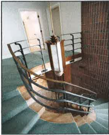
The Foyer Stairs
